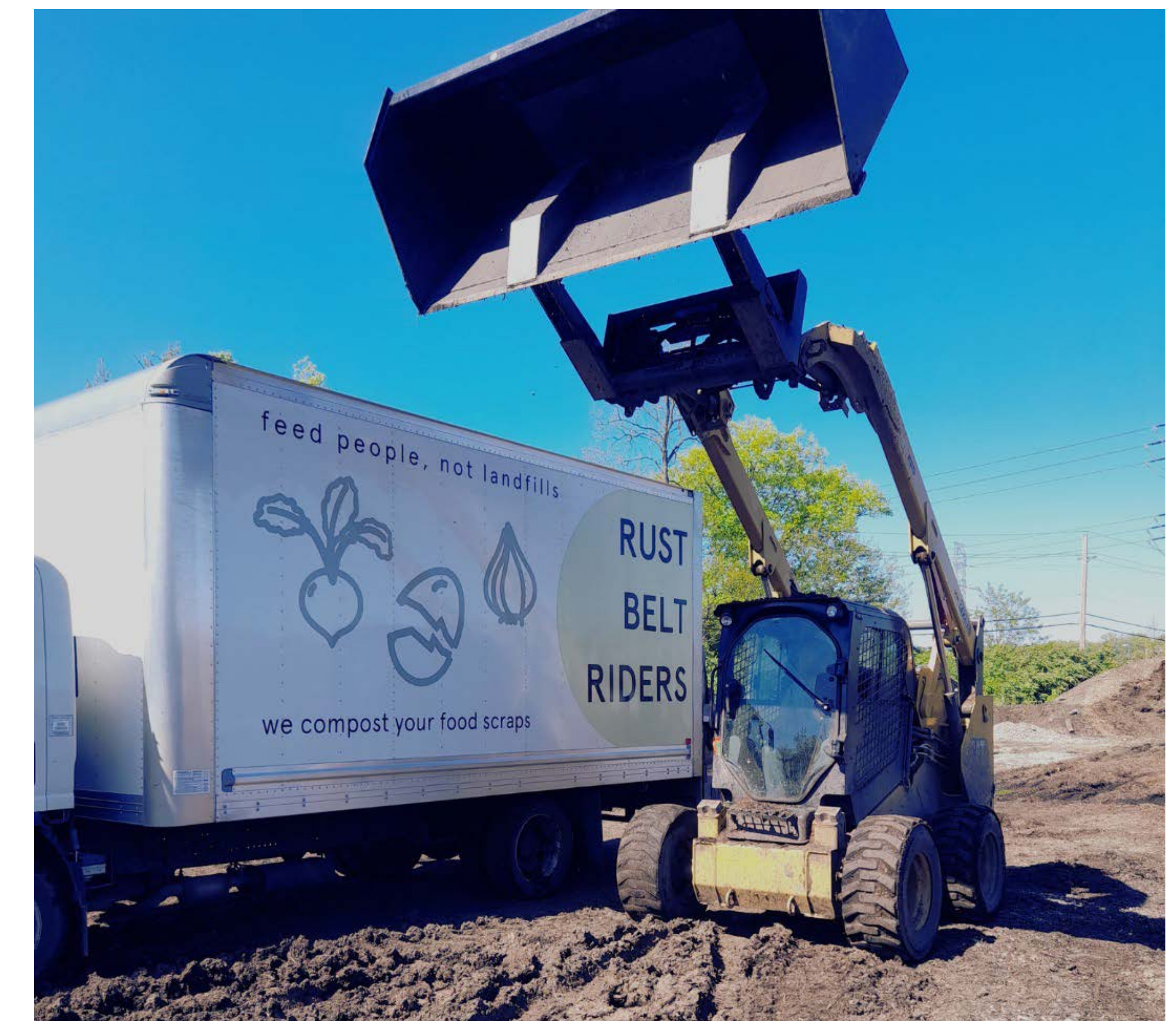
RBR food scrap processing site
