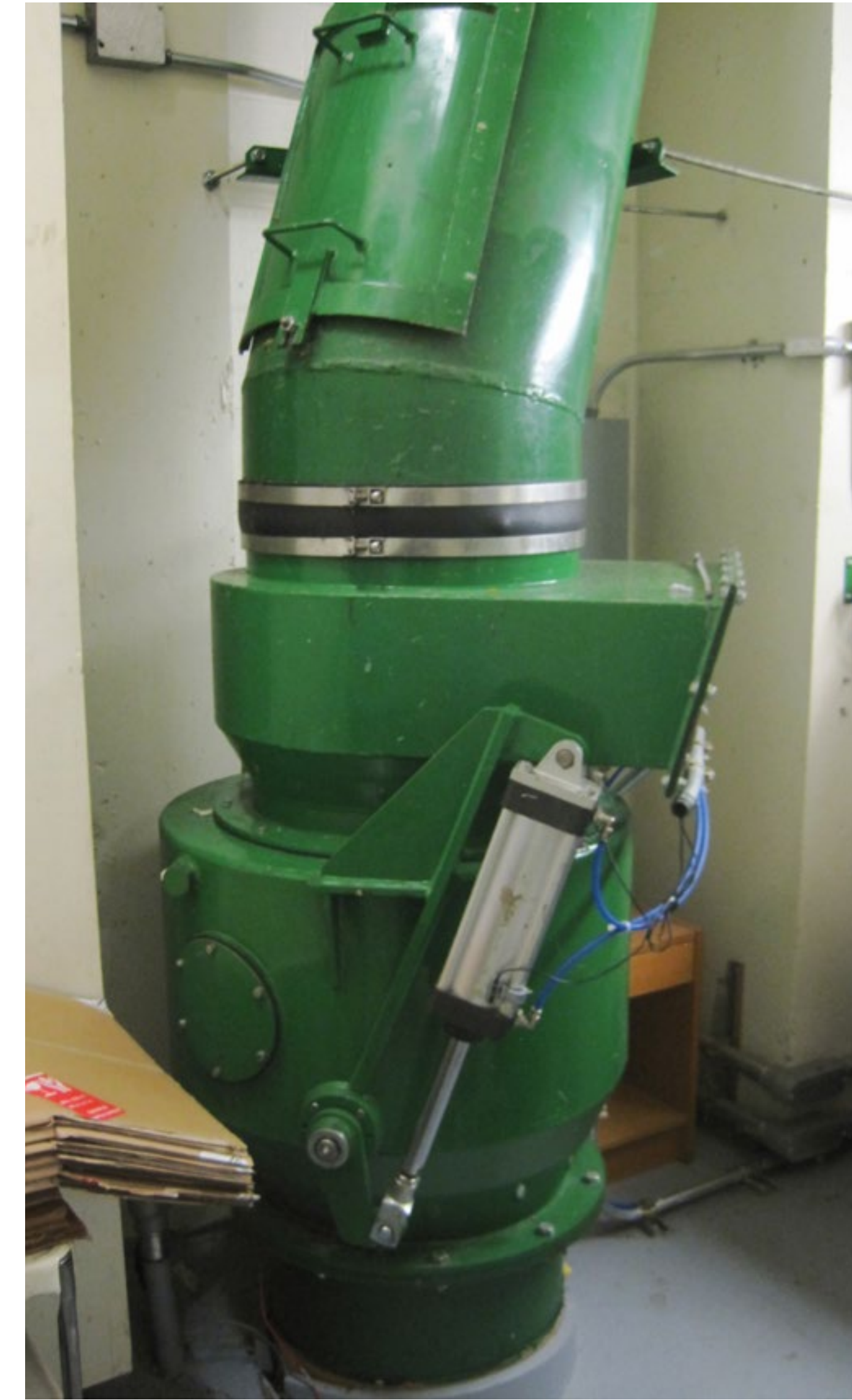
A valve in the building cellar at the base of a gravity chute connects to the pneumatic tube below; View inside the terminal (pneumatic tubes are painted red) including container moving equipment for 30 cu yd containers
