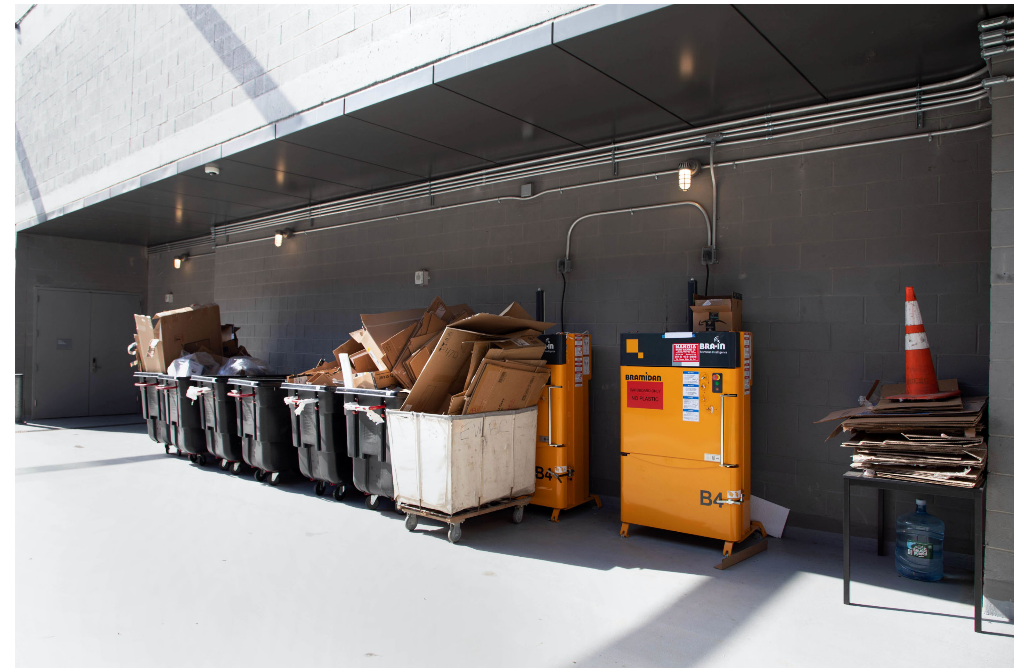
RoRos and balers in an enclosed yard at the rear of the building
